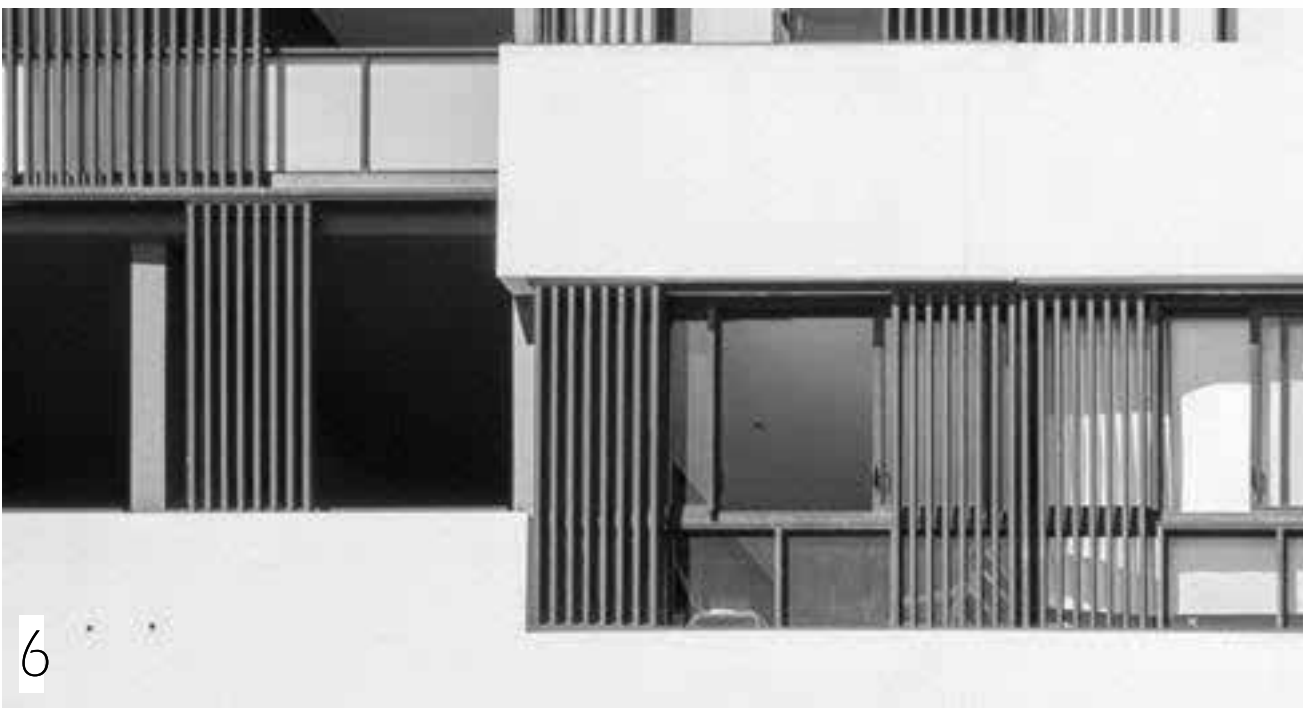
6 VERTICAL ALUMINIUM BATTEN SCREENS COLOUR - POWDERCOATED - DARK GREY
